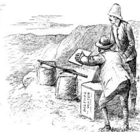
MacGregor's method, with sighting tube
